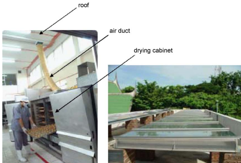
Fig. 61. (a) Schematic diagram of the solar-assisted drying system and (b) photograph of the drying cabinet inside the building and the solar collector on the roof of the same building [78].
