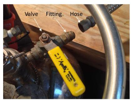
Figure 5.14. Close-up of the liquid ball valve and fitting.
