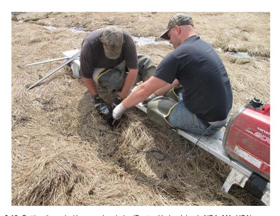
Figure 3.16. Cutting the rod with an angle grinder (Boston Harbor Islands NRA, MA, USA).
